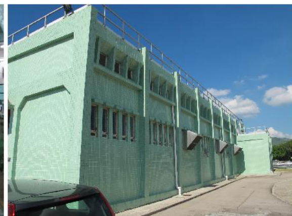
PHOTO 711: EXTERNAL VIEW OF BLOWER HOUSE (DATE TAKEN: 22 JULY 2016)
