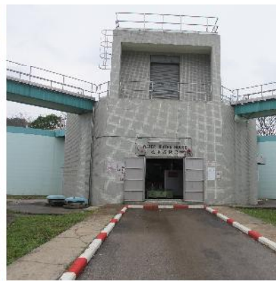
PHOTO 561: ENTRANCE OF WATER HEATER HOUSE (DATE TAKEN: 8 MARCH 2017)
