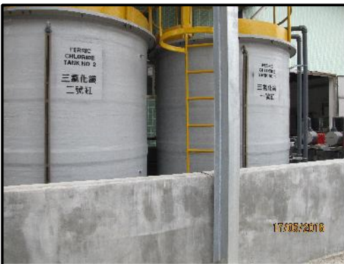
PHOTO 636: FERRIC CHLORIDE TANKS WITHIN DOSING FACILITY OUTSIDE THE SAS THICKENER HOUSE (DATE TAKEN: 8 MARCH 2017)
