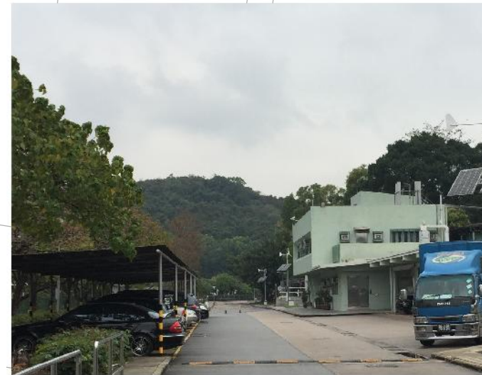
PHOTO 714: CAR PARKS AT YLSTW (DATE TAKEN: 8 MARCH 2017)
