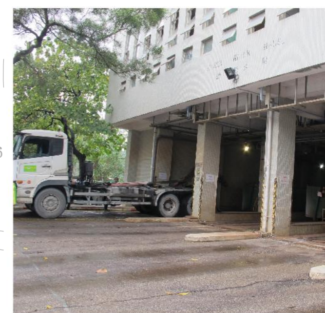
PHOTO 520: SLUDGE LOADING AREA OF SLUDGE DEWATERING HOUSE (DATE TAKEN: 8 MARCH 2017)
