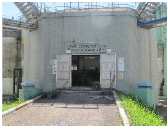
PHOTO 686: ENTRANCE OF METHANE COMPRESSOR HOUSE (DATE TAKEN: 22 JULY 2016)
