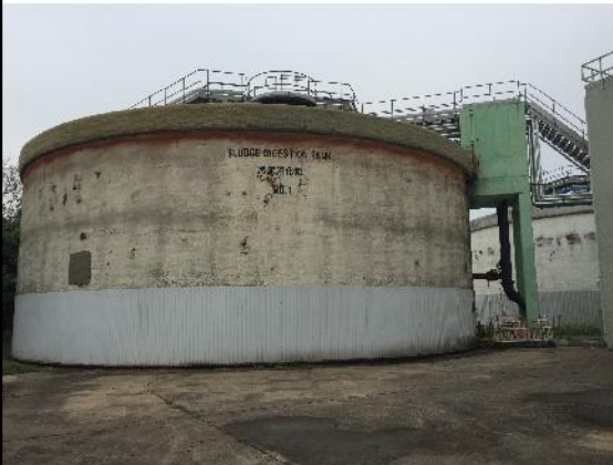
PHOTO 721: SLUDGE DIGESTION TANK (DATE TAKEN: 8 MARCH 2017)
