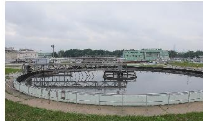
PHOTO 444: PRIMARY SEDIMENTATION TANKS (DATE TAKEN: 8 MARCH 2017)
