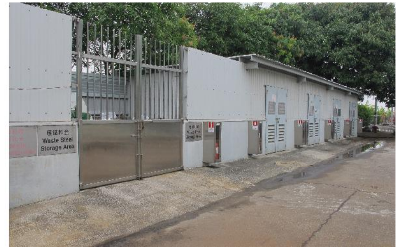
PHOTO 631: EXTERNAL VIEW OF WASTE STORAGE AREA (DATE TAKEN: 8 MARCH 2017)
