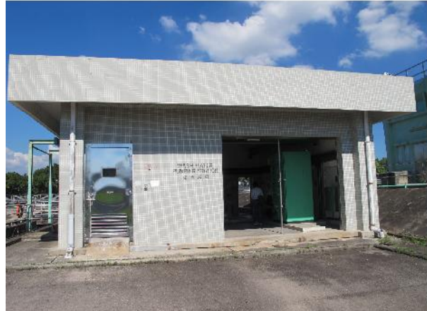
PHOTO 696: EXTERNAL VIEW OF WASH WATER PUMPING STATION (DATE TAKEN: 22 JULY 2016)
