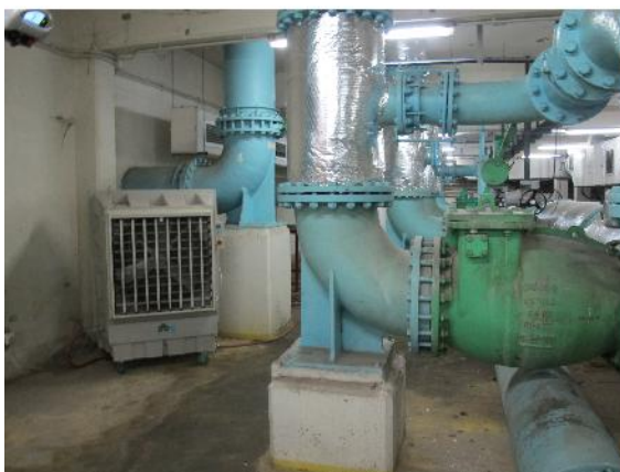
PHOTO 999: BASEMENT OF BLOWER HOUSE (DATE TAKEN: 22 MAY 2017)
