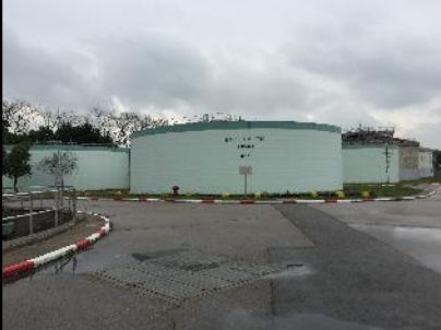
PHOTO 682: SLUDGE HOLDING TANK (DATE TAKEN: 8 MARCH 2017)
