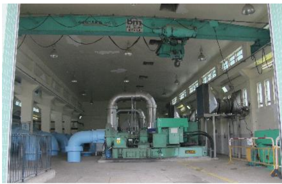
PHOTO 749: ENTRANCE OF BLOWER HOUSE (DATE TAKEN: 8 MARCH 2017)
