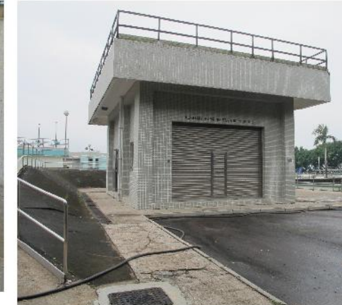
PHOTO 589: EXTERNAL VIEW OF AUXILIARY PUMPING STATION (DATE TAKEN: 8 MARCH 2017)
