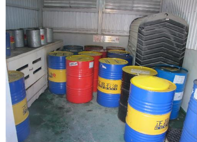
PHOTO 635: SPENT OIL STORAGE AREA (DATE TAKEN: 22 JULY 2016)
