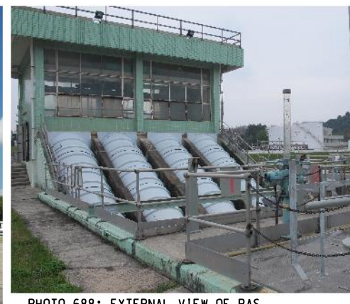
PHOTO 688: EXTERNAL VIEW OF RAS SCREW PUMP PUMPING STATION (DATE TAKEN: 8 MARCH 2017)
