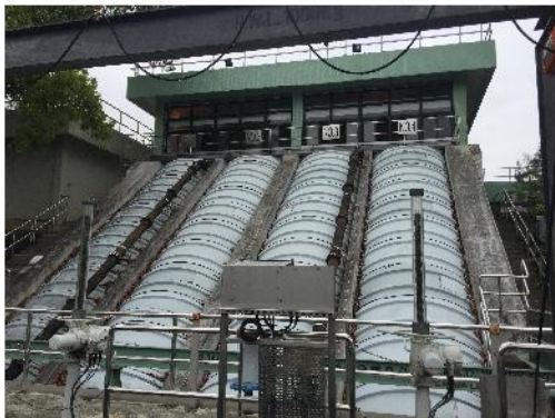
PHOTO 655: EXTERNAL VIEW OF SCREW PUMP PUMPING STATION (DATE TAKEN: 8 MARCH 2017)
