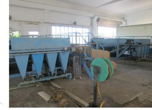
PHOTO 681: ABANDONED SLUDGE THICKENERS ON THE GROUND FLOOR OF SAS THICKENER HOUSE (DATE TAKEN: 22 JULY 2016)
