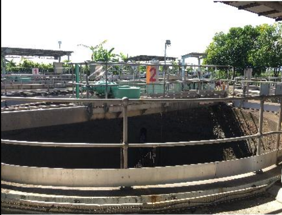
PHOTO 915: CONSOLIDATION TANKS (DATE TAKEN: 22 JULY 2016)
